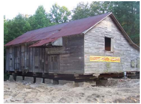
The mill is currently raised off its foundation
